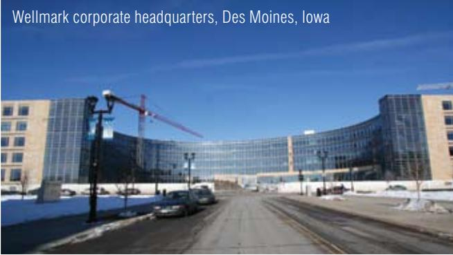
and installed the systems. The project features a custom-designed, laboratory-tested unitized stone and glass curtain-wall system that was engineered, designed, manufactured and erected by AWS. The large projects helped AWS weather the tough economic climate, according to company officials.
