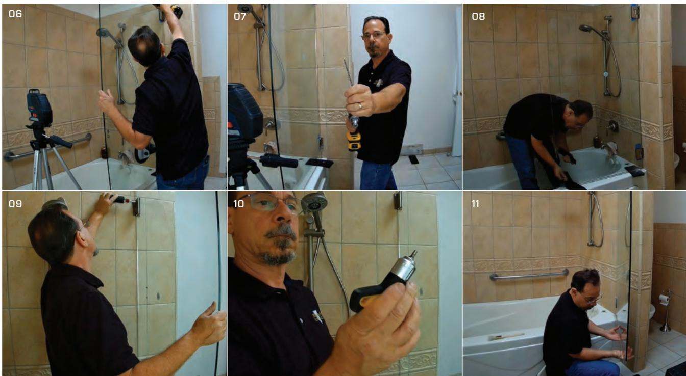
**06.** Line up the holes in the wall and hinge and insert a screw. Now that the first screw is in place, the installer is free to work on securing the remaining screws. Use the laser to line up the hinges to ensure they are plumb.
