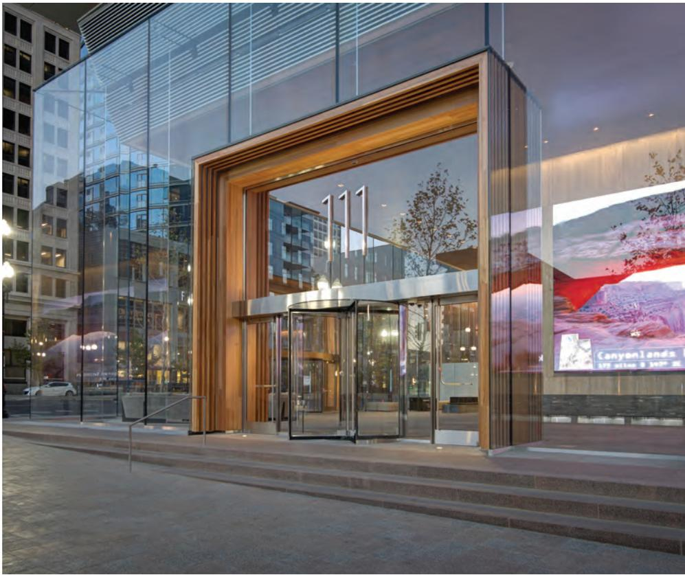
111 Main in Salt Lake City features a lobby enclosed in 35-foot-tall, ultra-clear, low-iron structural glass. The glass is laminated glass with SentryGlas from Kuraray. Photo by Steel Encounters.
