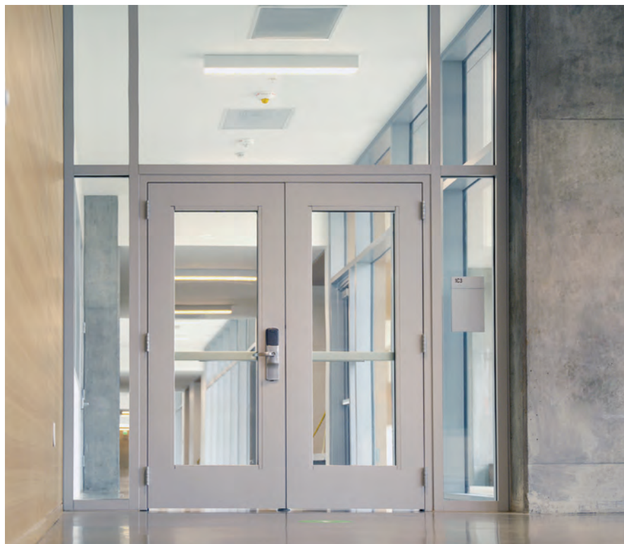
1-hour Fire Resistive Wall with SuperLite II-XL 60 in GPX Architectural Series Framing and Full-vision 60 Minute Pair Doors with SuperLite II-XL 60 in GPX Builders Series Temperature Rise Doors. Photo by SAFTI FIRST.
