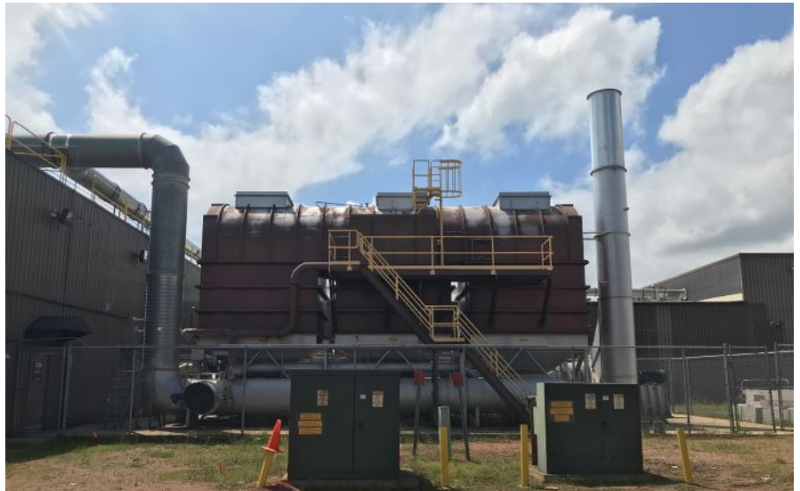
Linetec uses its regenerative thermal oxidizer, pictured, to destroy volatile organic compounds. VOCs are created in the painting process; the company captures all VOCs, and destroys 99.4 percent in the regenerative thermal oxidizer, according to the company.
