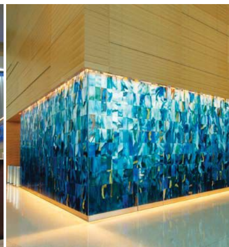
A 160-foot wide, 10-foot high glass art installation wraps around four walls at the CalSTRS Headquarters in West Sacramento, California. The piece consists of mouth-blown glass that is slightly milky, painted with vitreous enamels that are fired onto the glass, then laminated to mirror. The mirror reflects the ambient light in the space through the mouth-blown glass. Paul Housberg of Glass Project, glassproject.com , created the glass; HOK, hok.com , was the architect.
