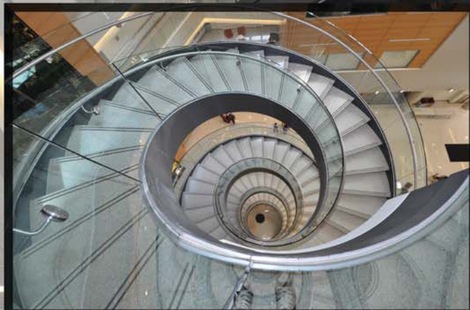
Self-supporting, helical staircase at Drexel University.
