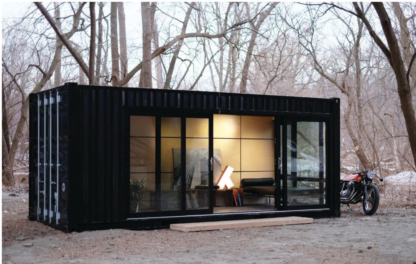
The Glasshaus Container from Glasshaus Living, [glasshausliving.com](http://glasshausliving.com), features a 16-foot glazed opening in a repurposed shipping container, creating a serene and quiet portable office space. The container features tilt and turn windows and a bi-parting door with Rehau vinyl profiles, supplied by Euro Vinyl Windows and Doors Inc. This photo was the third in a series that documented the installation of the glazing systems on the steel container.
