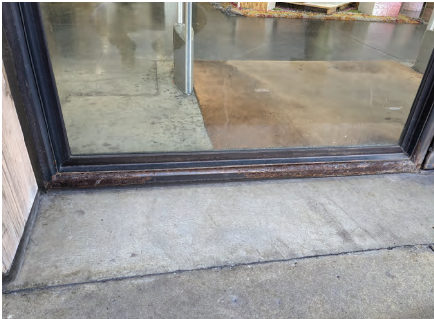
Example of finish damage on a commercial building due to chemical moisture.
