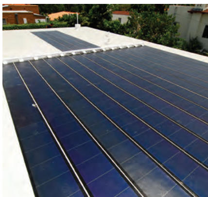
Thin film flexible PV panels on rooftop. Photo Ken Fields, Creative Commons
