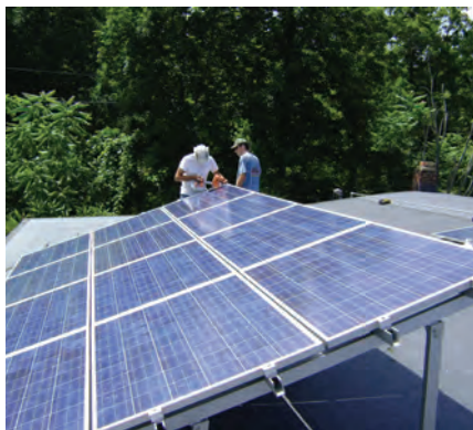
Tilt-up solar PV module array on rooftop. Photo Lucas Braun, Creative Commons
