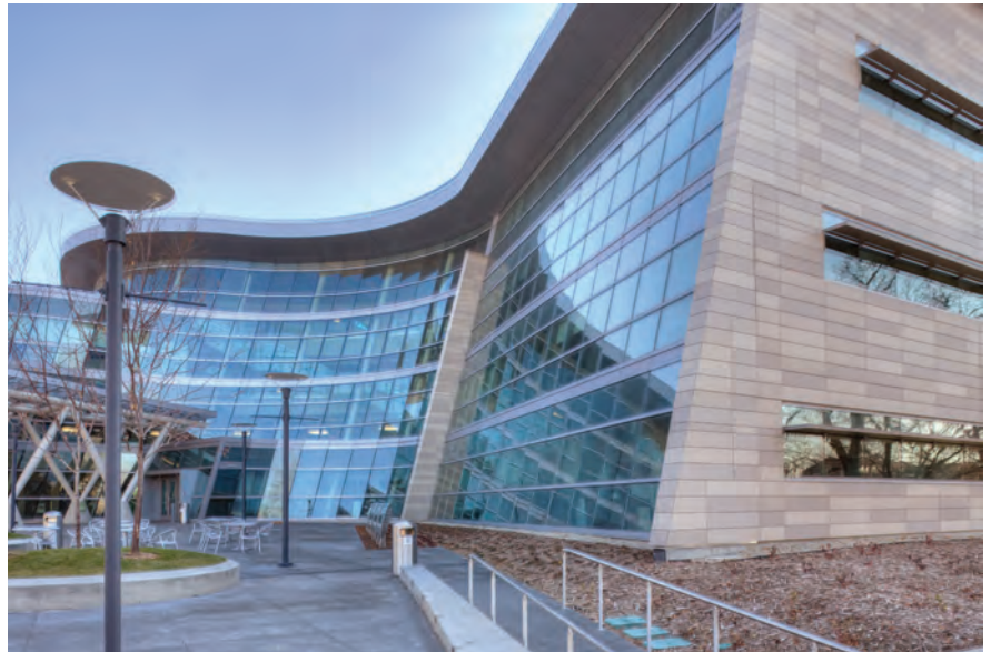
Example of laminated glass curtain wall at Salt Lake City Public Safety Building. GSBS Architects, Photo by Wayne Gillman
