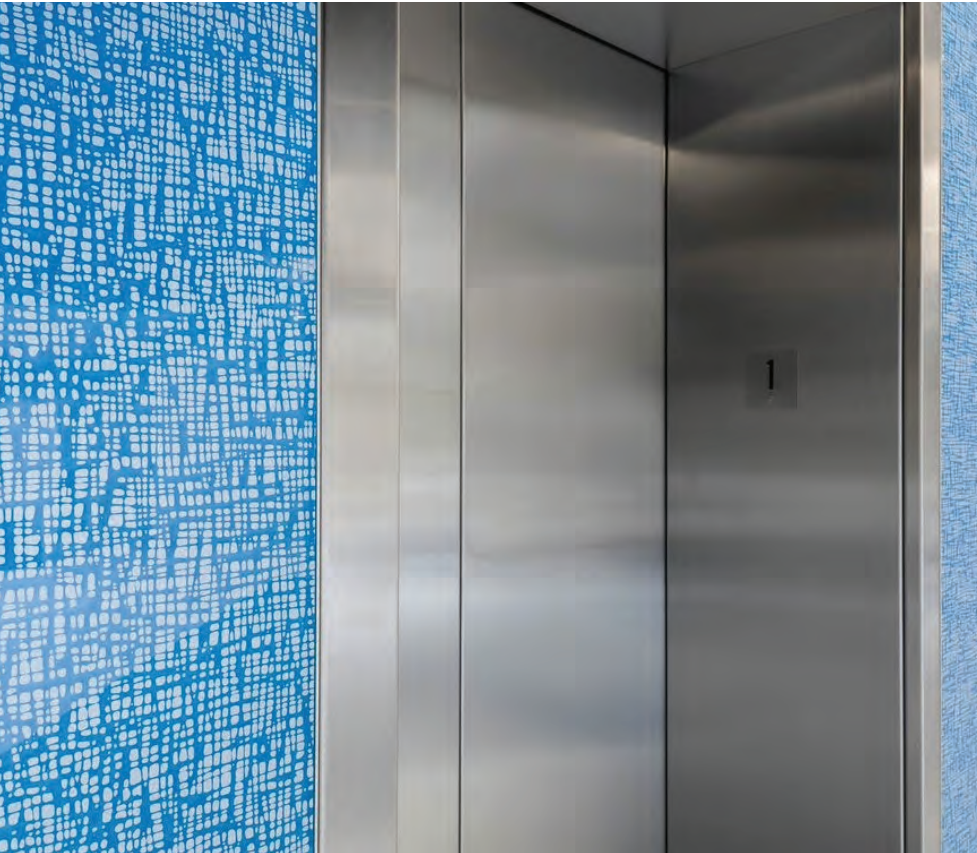
Project incorporating both ceramic frit direct-to-glass printing for the design with a custom blue water-based silicone back-painting for this opaque wall cladding application.
