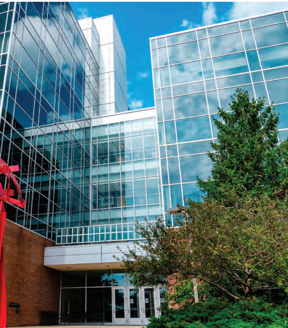
Ubiquitous Energy transparent solar window project at Michigan State University in East Lansing, Michigan. Photo courtesy of Ubiquitous Energy.
