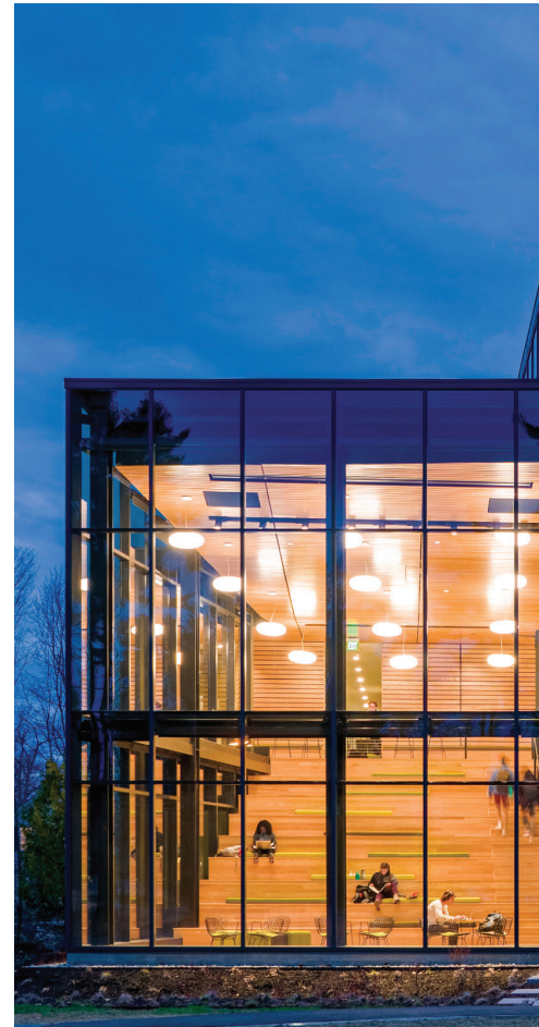
Above: Fireframes SG Curtainwall Series with Pilkington Pyrostop glass firewall by TGP was used for the stairwell exterior façade of the Roux Center for the Environment at Bowdoin College in Brunswick, Maine. Photo courtesy, TGP, © Jeff Goldberg/Esto.
