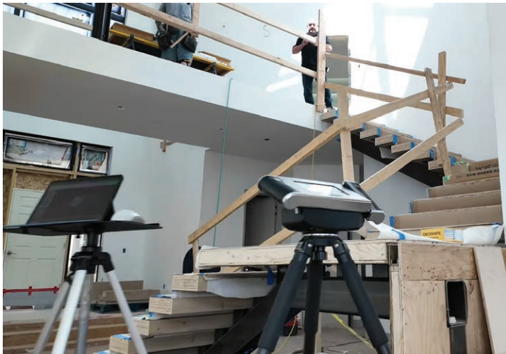
REDLINE TEMPLATES USES LASERS ON THE JOBSITE TO ENSURE PRECISE DIMENSIONS AND MEASURING.
