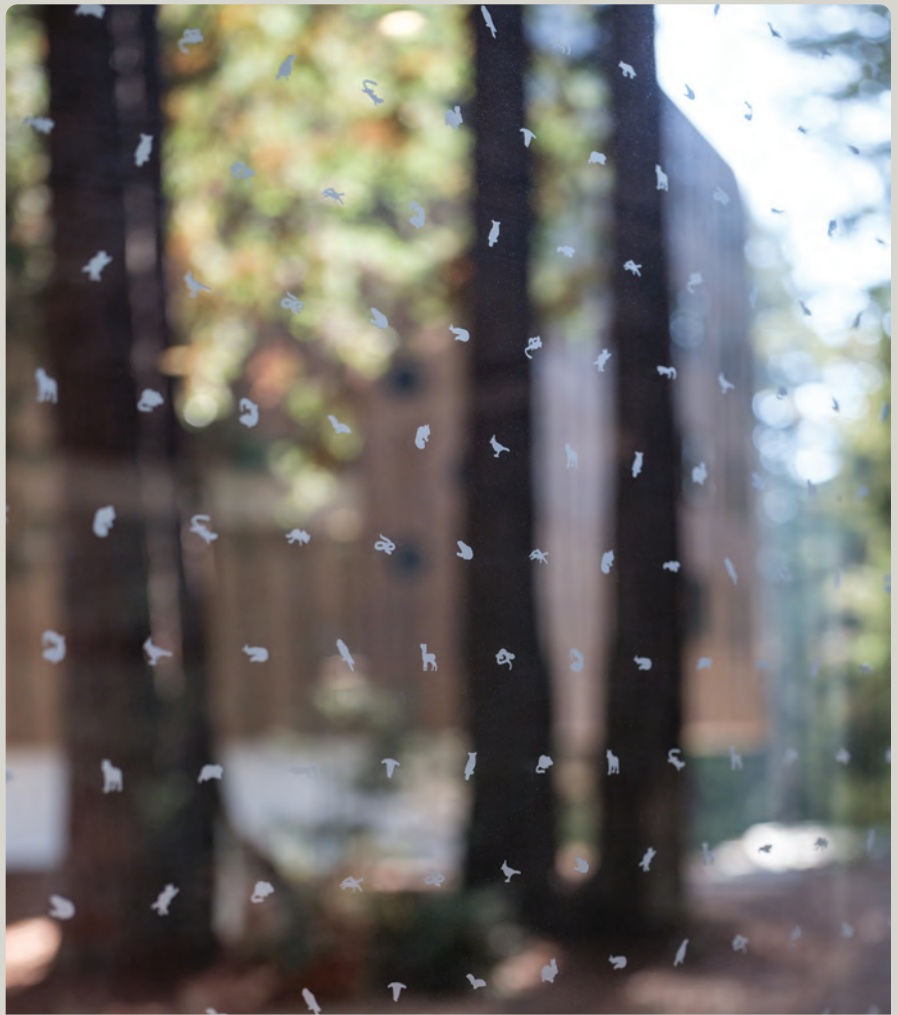
Skyline worked with architecture firm Studio Gang to create a unique design for this bird-friendly glass. While the pattern may appear as dots, it displays small silhouettes of animals native to the area around the project, Kresge College at the University of California. Phot by Jason O’Rear Photography.
